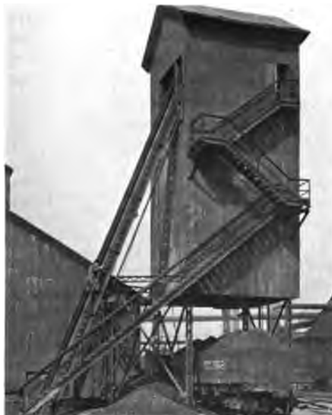
Fig. 3. Structural Steel Stairway for Coal Hoist.†
